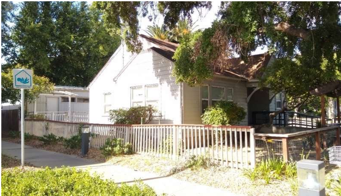
East façade, looking west. The portable building is visible at left. ESA, 2022.
