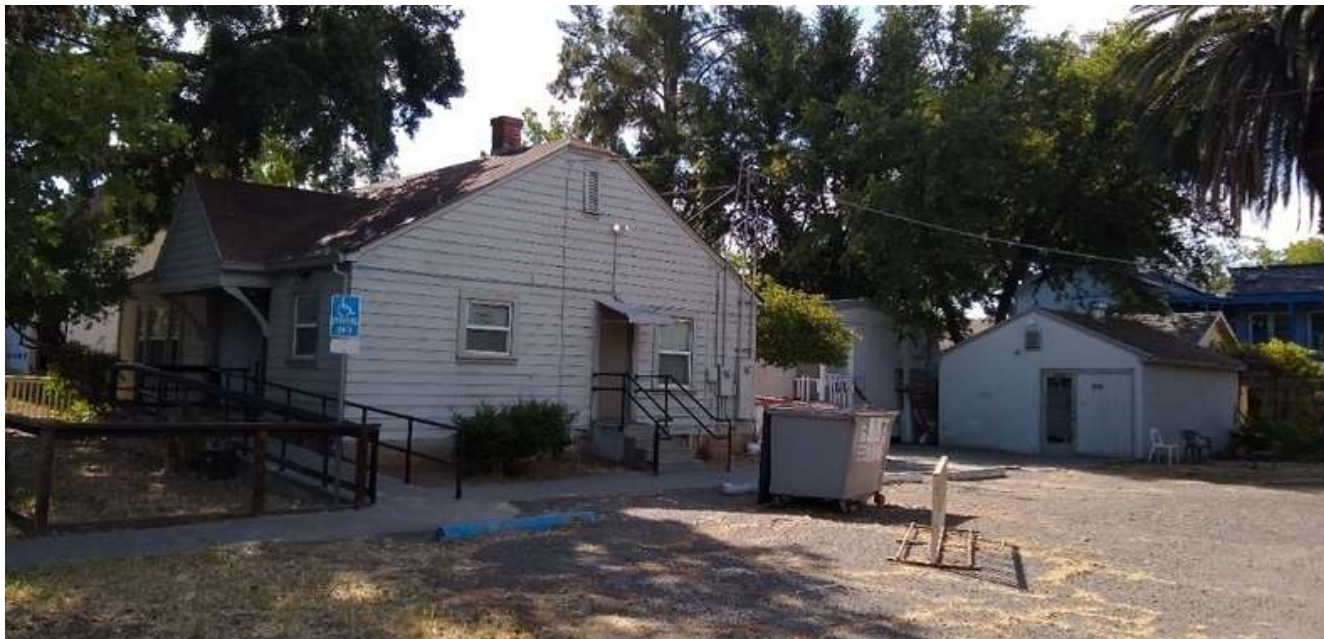
West (secondary) façade, looking east. The two rear buildings are visible at right. ESA, 2022.
